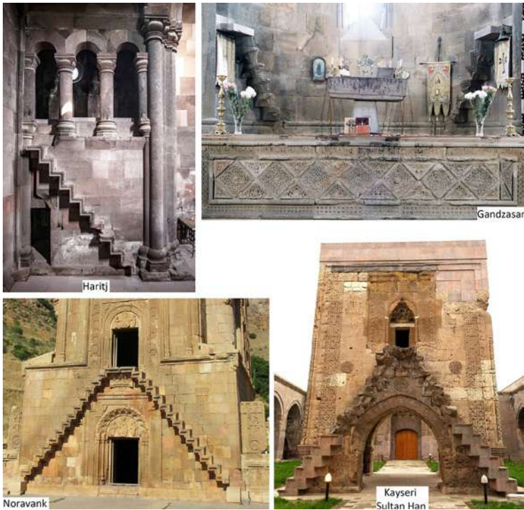
Figure 16 Pairs of corbelled staircases on Armenian monuments (13th-14th c.) and on the 'kiosk-mosque' of Kayseri Sultan Han (c. 1230-36). Photos of Haritj and Kayseri © H.H. Khatcherian; of Gandzasar © Z. Sargsyan; of Noravank © Author
