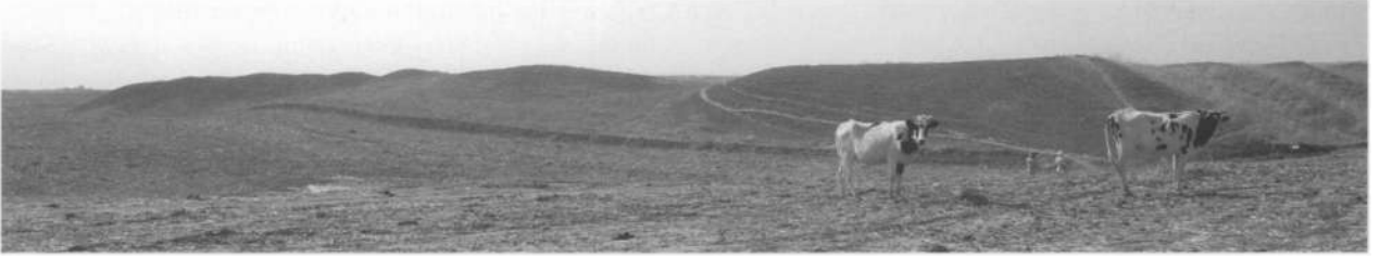
Fig. 31. Fort 4 (like the other forts on the Gorgan Wall) forms a substantial platform, here the small side seen from the south-east. Note the human scales (between the cows) in close vicinity to the fort.
