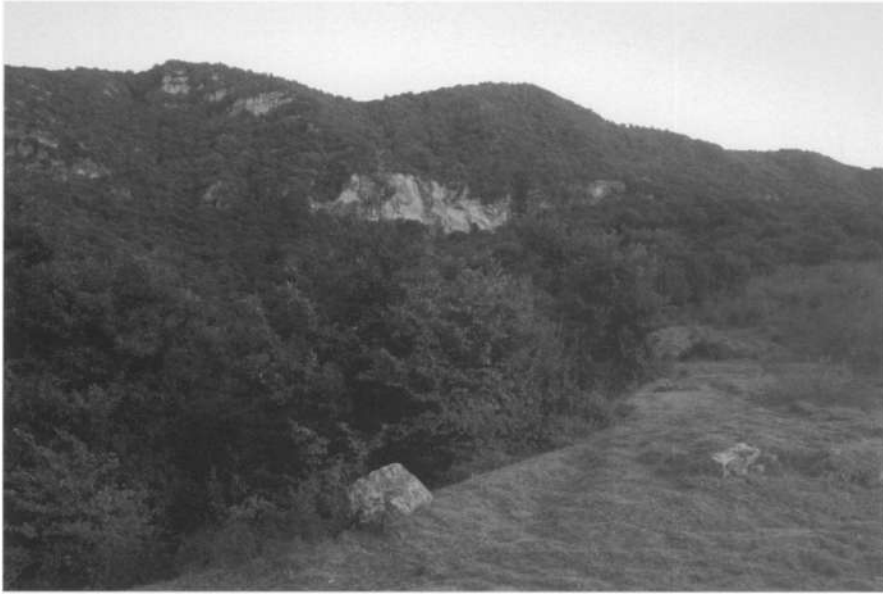
Fig. 5. The Great Wall of Gorgan, marked by a scatter of fragments of the typical bricks, follows the grass-covered ridge in the foreground, overlooking a deep valley to the left, and extends to the vicinity of the vertical rock face in the Elburz Mountains in the background (or possibly beyond).
