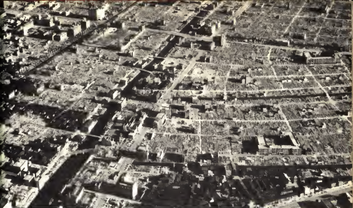
The residential section of Tokyo after the terrible fire-bomb raid. Only large modern buildings were strong enough to withstand the explosions and fires.
