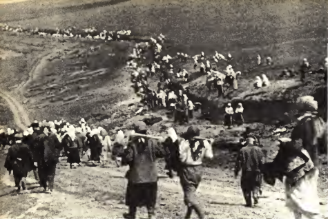
Moscow factory workers turn out after hours to dig antitank ditches. The people of the capital were required to build four defense lines; one beyond the city limits, a second at the city border, and two within the city itself.
