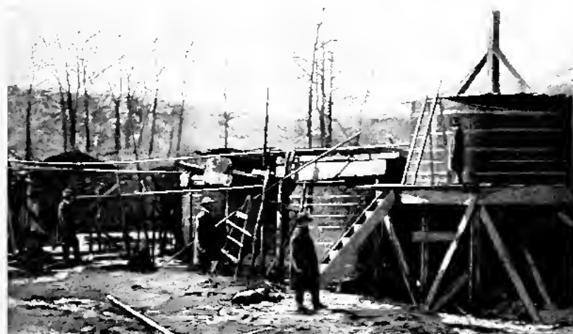
WOODEN TANKS FOR STORING OIL
